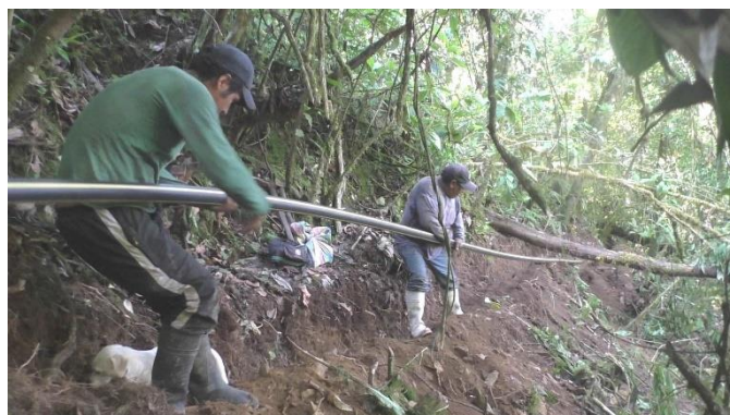
The 3 km-long water hoses were buried 30 cm deep in challenging terrain.
