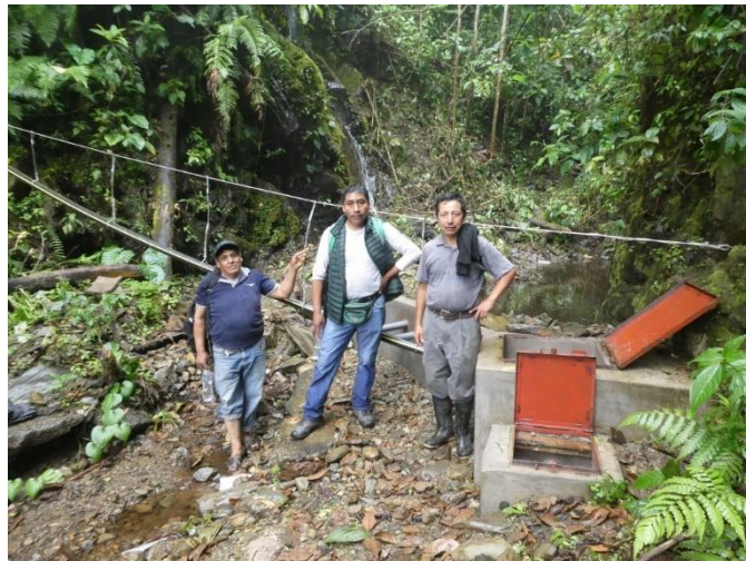
Water chamber. From here, the water flows for approx. 3 km through hoses and pipes to the agricultural areas.
