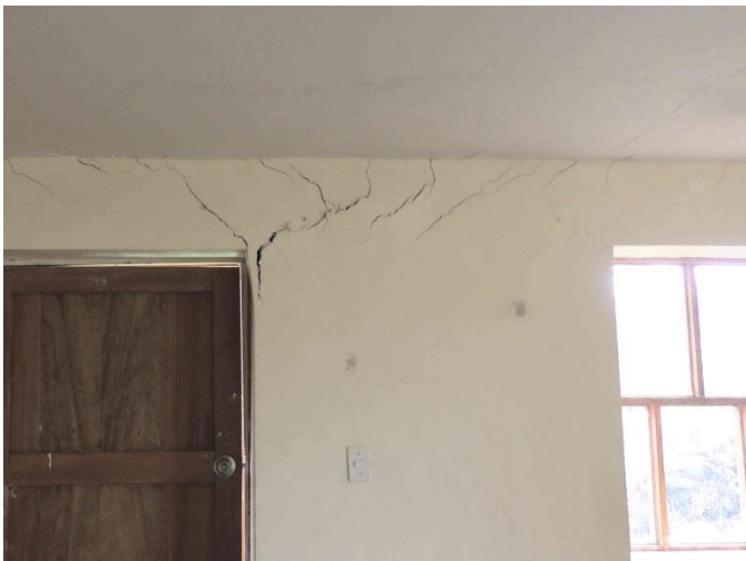
Condition of the interior walls before renovation.
