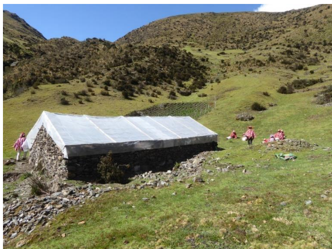
Exterior view of one of the greenhouses we built. The UV-resistant roof film has a service life of approx. seven years.
