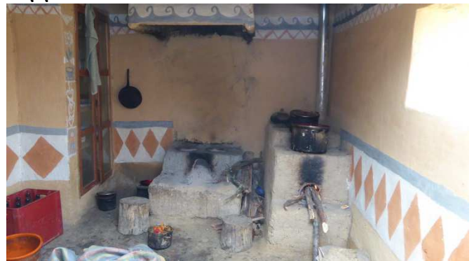
Improved kitchen oven with chimney and cast iron pipes within the oven. The smoke is lead outside.
